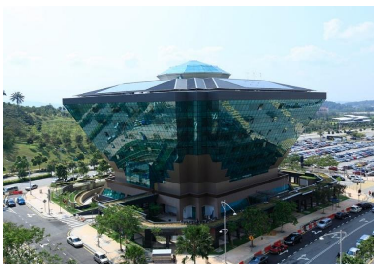
Figure 6. ST Diamond Building (Photo credit: Original)
