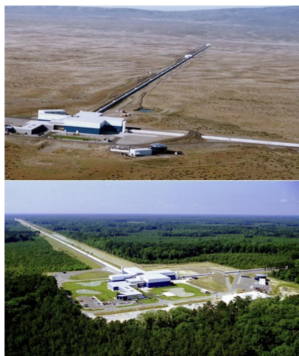
Fig 1. Two photos of the LIGO observatories showing an overview of the buildings [7].
